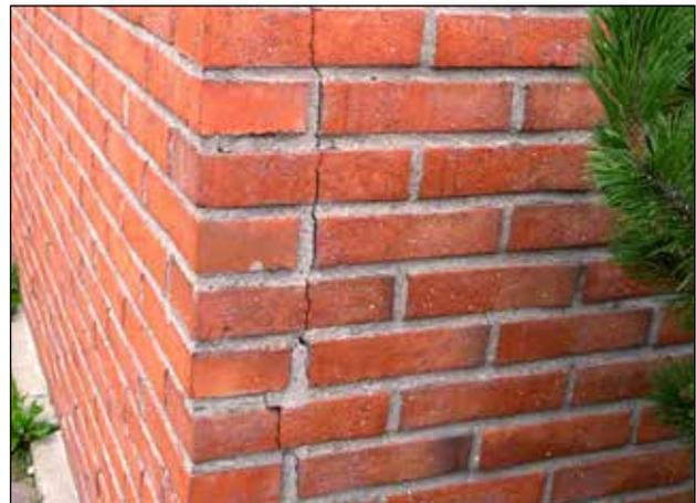
*An example of a brick cavity wall expanding over the corners as a result of the horizontal joints forming long pressure bars.*
