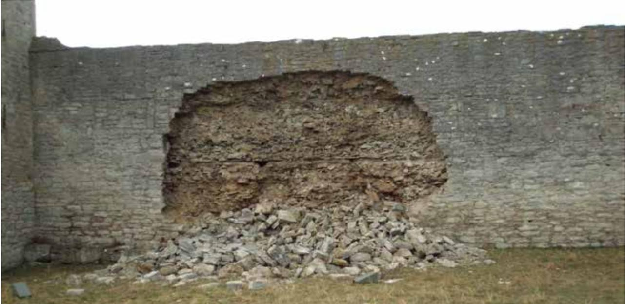
*An example of a wall which was repointed with a sand-rich, non-elastic mortar.*
