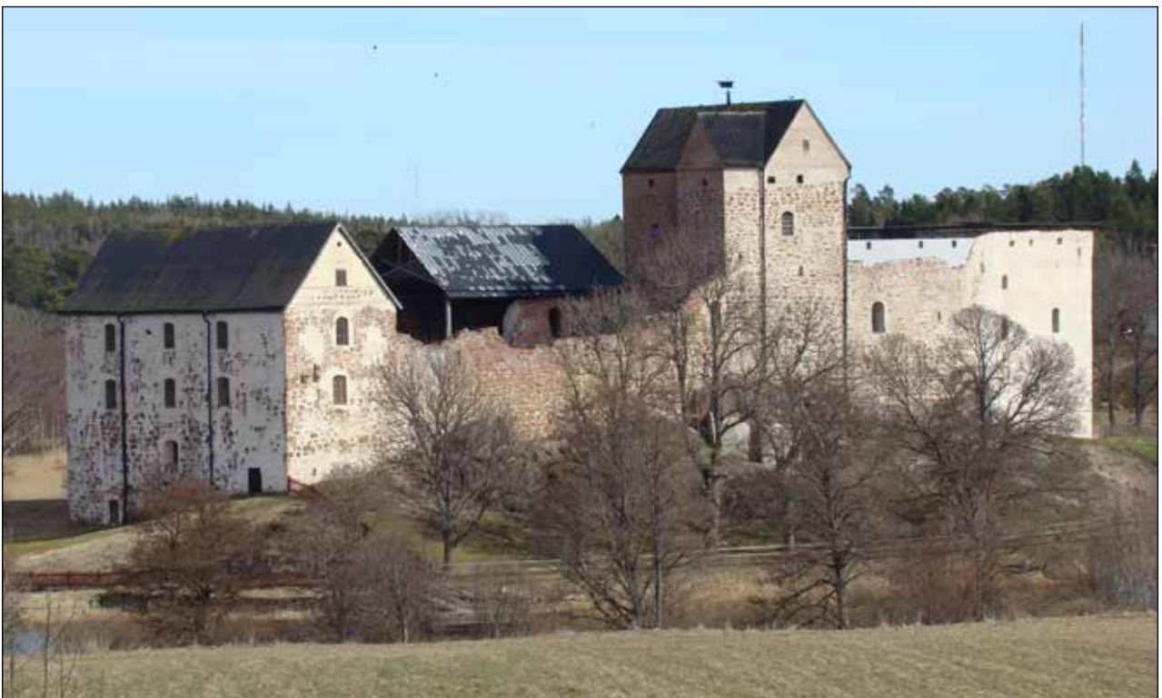
Elastic joints permit the use within certain limits of larger and smaller building stones without these affecting the neighbouring stones.
