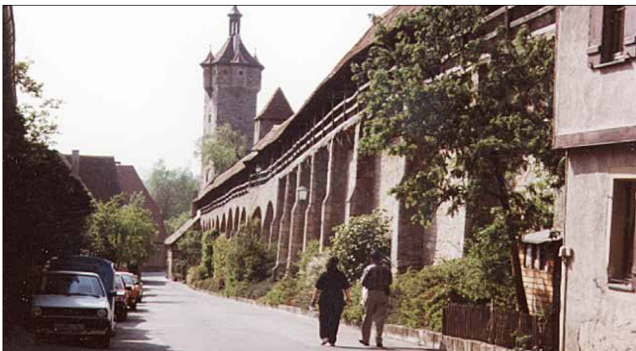
Elastic masonry which is protected by a peacetime roof.
